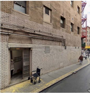
Doyer street resi. entrance
